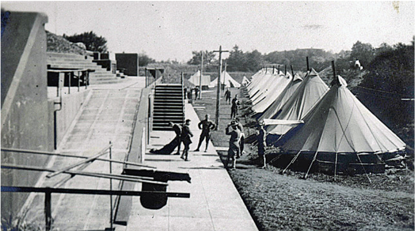
This Photo reveals the interior of the old earthworks as it appeared in 1917-18. In view is Battery Freeman which had two 6-inch guns and one 3-inch gun. It was built inside the parapets of the earthworks, not an uncommon thing to do. The tents in the background are behind the 3-inch gun. The space was used as a cantonment for the 65 th CAC while waiting to be shipped out to France.
